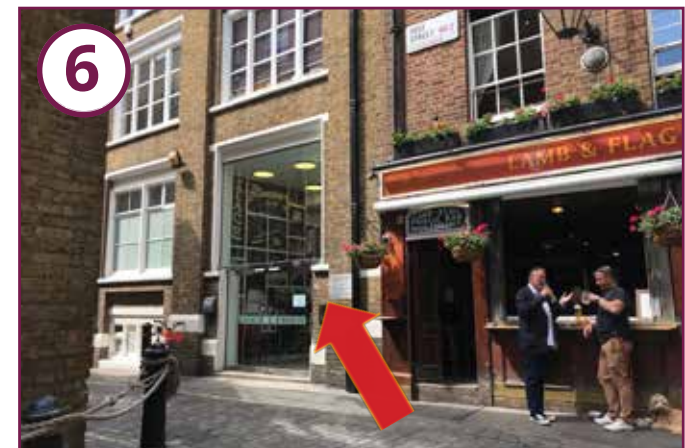
The office is next door to the Lamb and Flag pub. Entry is via the double glass doors. To enter, press the intercom to communicate with our reception team.
